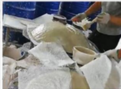
④ GROUTING ④灌浆
